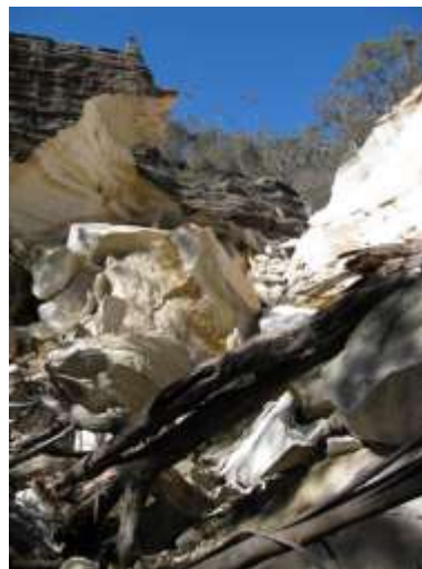
Cliff collapse in ‘80s on left, just 1 km west of Maiyingu Marragu, over 100,000 tonnes (note figures at base of cliff). Cliff Collapses in Baal Bone Colliery (right) in 2009).
